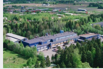
PEIRON OY STEEL FOUNDRY KOKEMÄKI, FINLAND
